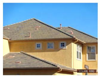
Tile roofs are designed to last the life of a community. However, the underlayment (waterproof membrane underneath the roof tiles) can be subject to deterioration and failure through time. The timing and rate of failure is difficult to predict and can vary significantly from one project to another depending largely on the quality of the original design and construction (materials and installation), exposure to outside influences (climate, foot traffic, etc.) and the level of routine maintenance.
